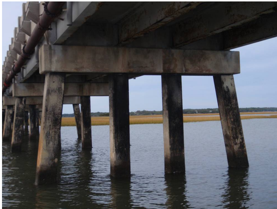
Photograph 5. View of Bent 29, Typical of Bents 30 through 32, 35 through 39, 42 through 44, 45 through 47, 50 through 52, 55 through 58, and 61 through 63.
