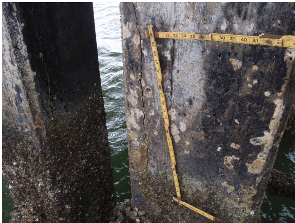
Photograph 11. View of a Typical Vertical Crack in a Pile.
