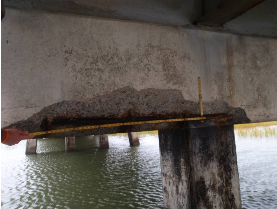
Photograph 13. Spall in west face of Bent 63 cap.
