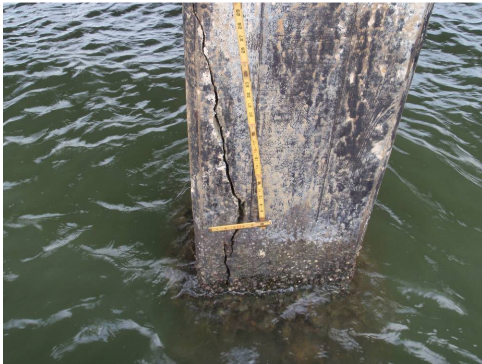
Photograph 12. View of Crack in Pile 1 at Bent 61. Typical of larger cracks.
